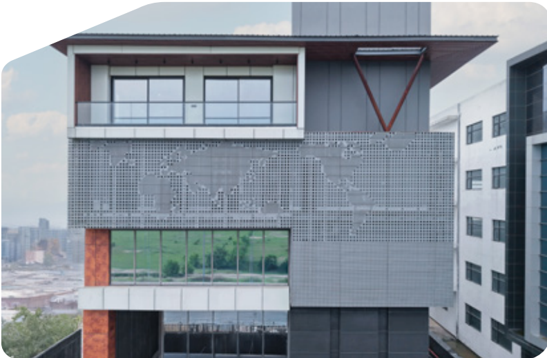
Office Building, Noida | System: Interlocking panel with Perforation | Finish: QUARTZ-ZINC
