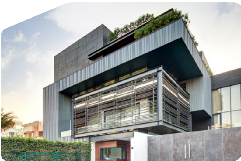
Individual Residence, Gurugram | System: Standing seam panel | Finish: PIGMENTO blue
